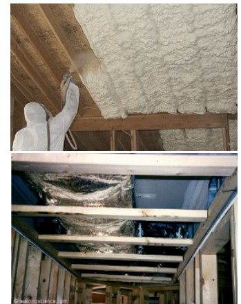
Top: Spray foaming roofline. Bottom: Dropped soffit.
