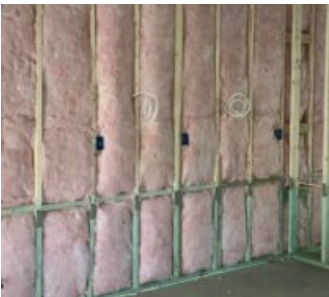
Grade 1 insulation installed mid-construction.
