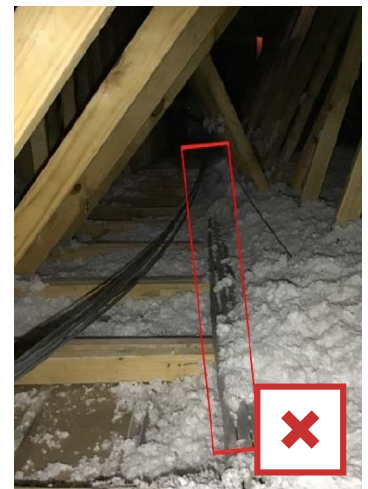
Lack of a rigid air barrier enables insulation to spill over from insulated areas (above units) to uninsulated areas (over breezeways).
