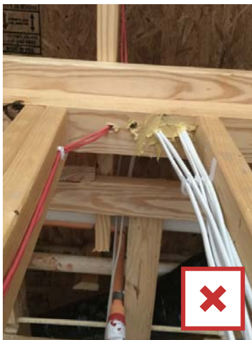
Unsealed penetrations through the top plate.
