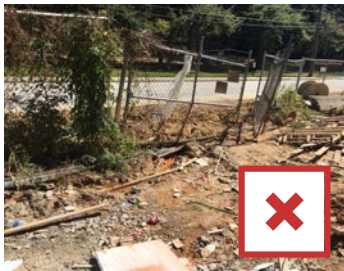
Poorly maintained silt fencing around the construction site perimeter.
