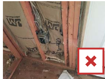
Poorly installed fiberglass batts.
