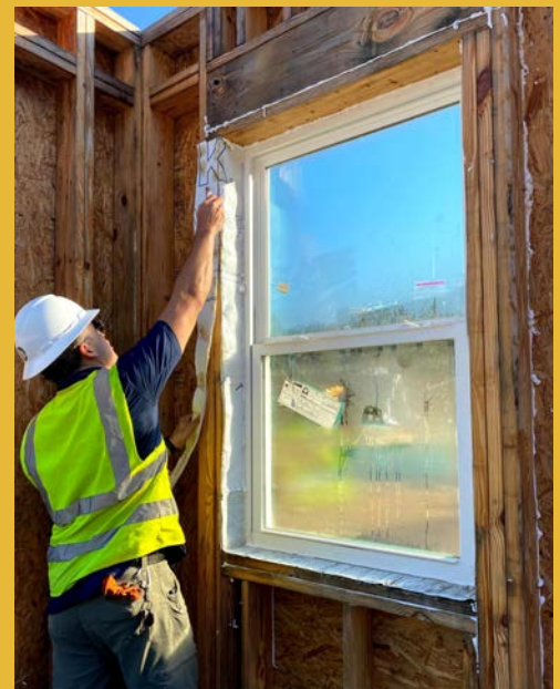
SK verifier assesses air sealing measures around windows.
