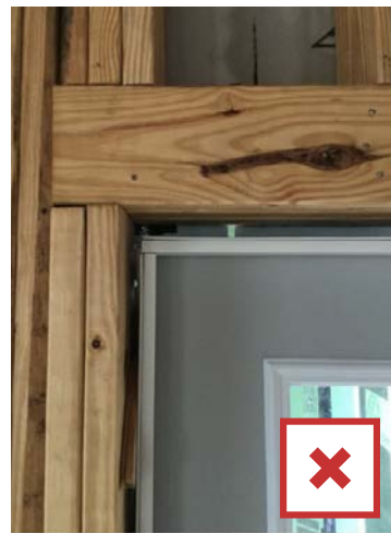
Visible gaps between wood frame and window lead to air leakage and water intrusion.
