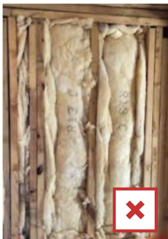
Compressed insulation leads to uneven distribution and R-value effectiveness.
